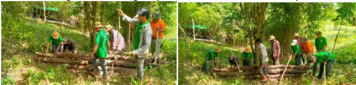
Figure 105. Practicing Leaky Weir Installation at Takhes Meanchey
