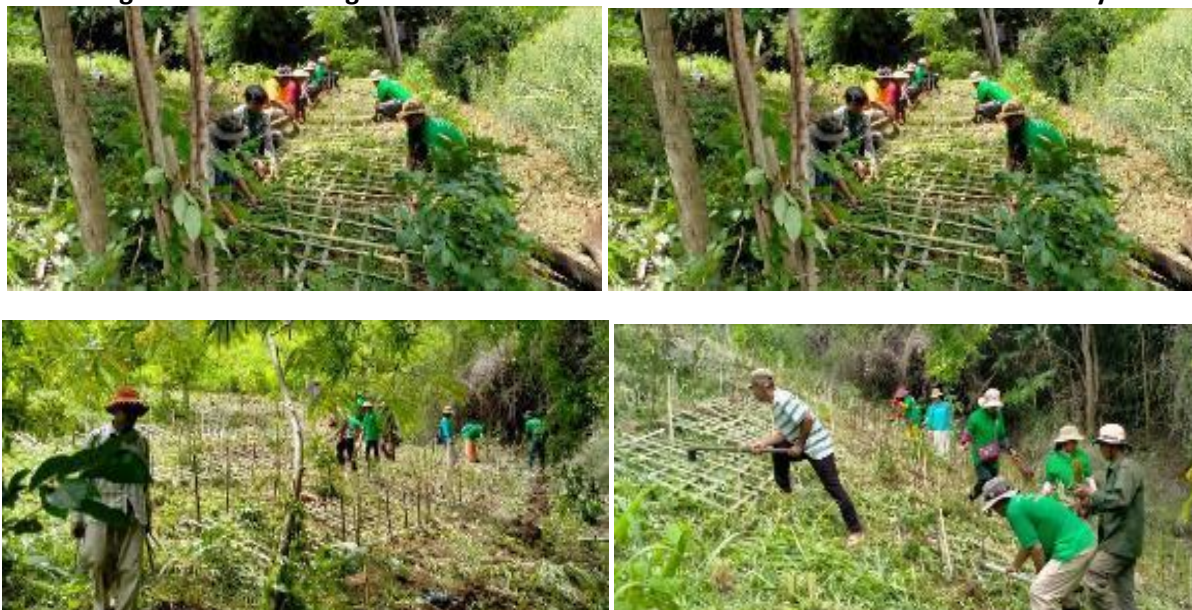
Figure 104. Practicing Soil Erosion Control Measure Installation at Takhe Meanchey
