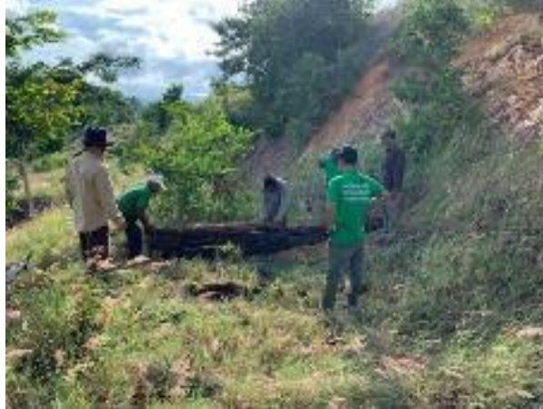
Figure 102. Practicing Brushwood Leaky Weir Installation at Anakut Koma Samaki
