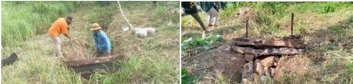
Figure 108. Practicing Leaky Weir Installed at Dontret Restoration Site
